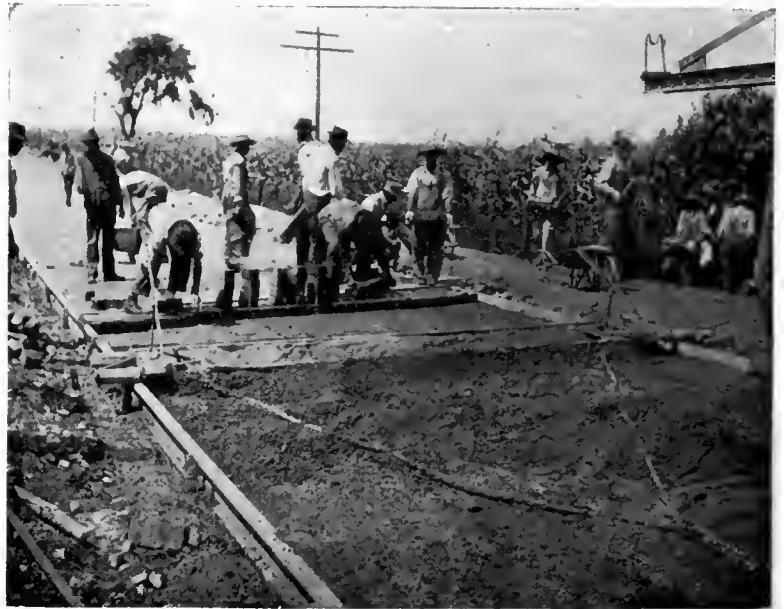
Fig. 4—Laying brick, Paris, Ill.
